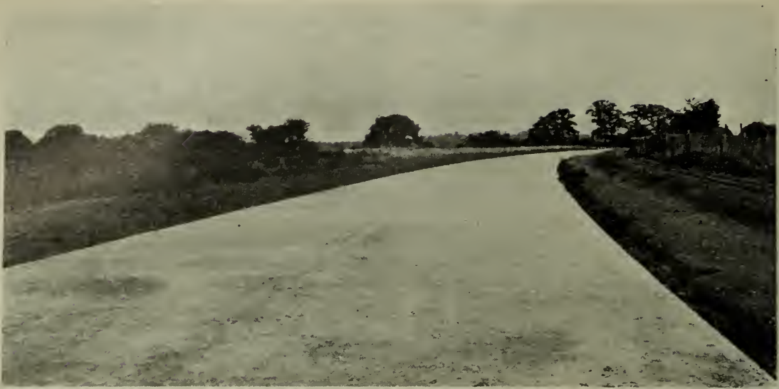
NEW REINFORCED CONCRETE ROAD AT WILLESDEN.
